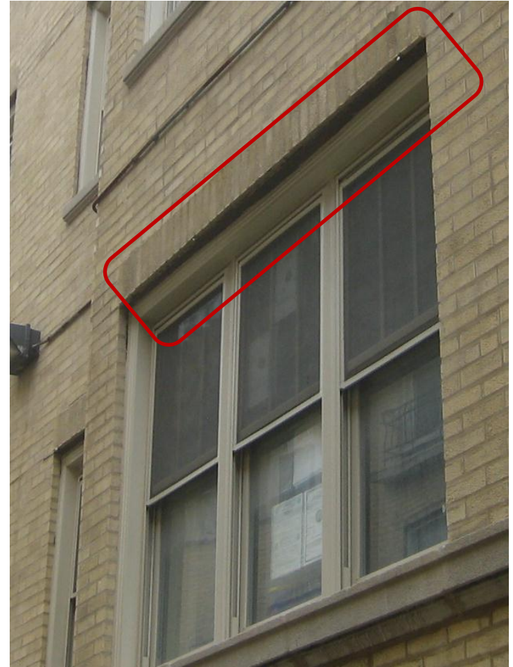
New lintel in place
