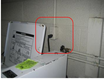
GFCI outlet needed at washer/dryers Also required at all kitchen & bathroom outlets
