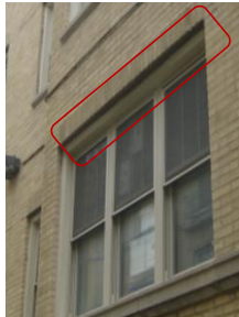
New lintel in place
