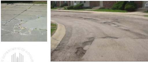
Patch repairs, full replacement, seal coat... Silicate bids from a professional as necessary.
